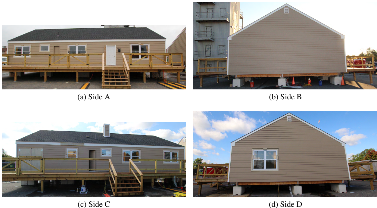
Figure 2.1: Representative exterior photographs of the four sides of the experimental structures.
