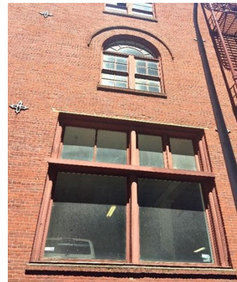
Note tie plates in place as well as the arched spandrel above the upper window. A lintel can be noted above the double windows to provide reinforcement and serve as a small header.
