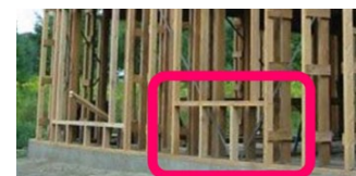
Example of platform construction.
