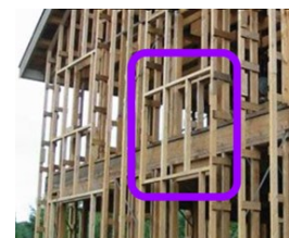
Example of balloon frame construction.
